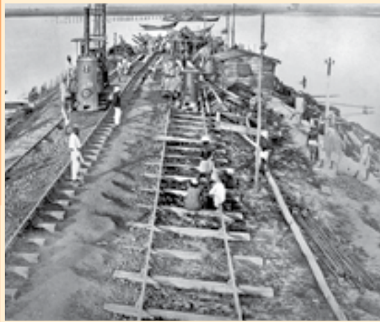
Under British rule, thousands of miles of railroads were built across India. Here, workers build the East Bengal Railway around 1870.
